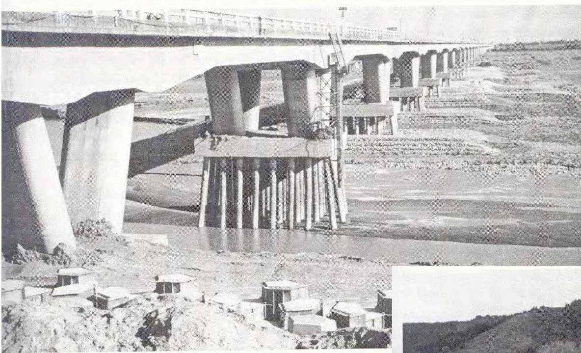
Figure 4.8. Degradation exacerbated by sand extraction for Republic of China.
