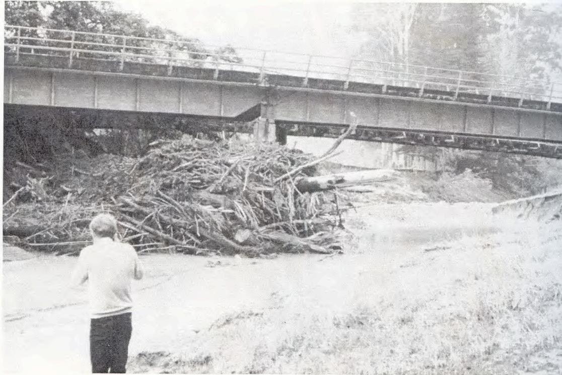
**Figure 1.5.** Floating debris accumulation at a bridge pier, bridge on Tauwhareparae Road over Mangaheia River, New Zealand, Cyclone Bola, 1988.
