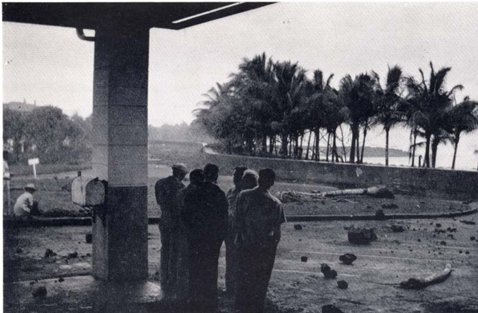
Figure 1b. Sea wall at the Puu Maile Hospital, Hilo, after the 1 April 1946 tsunami. Photo by Mrs. Pearl Welsh (Plate 30a in Shepard, Macdonald and Cox, 1950, p. 521)
