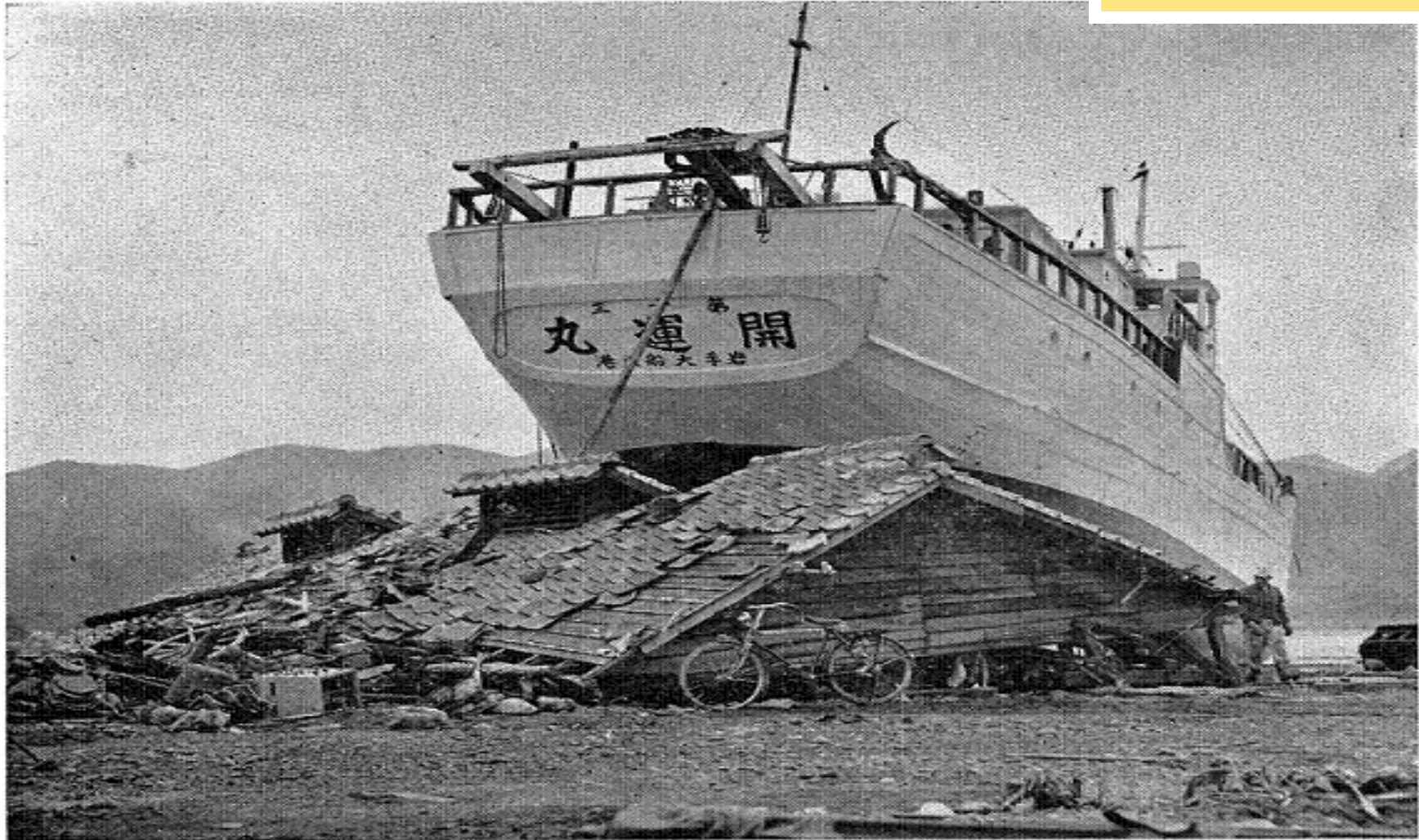
Fig. 21. House crushed down by a fishing boat at Ofunato, Iwate Pref. (Courtesy of Asahi Shimbun.),
