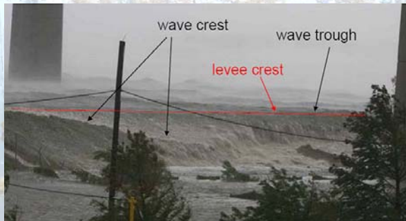
Surge over-crests levee under Paris Road Bridge during Hurricane Katrina
