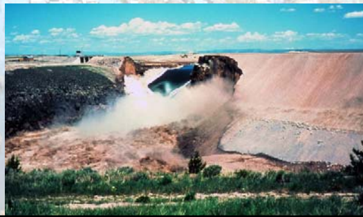
Failure of Teton Dam, 1976
